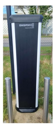
For both chargers the cable will lock into the vehicle and charger once charging is initiated and will unlock when you end the charge.
